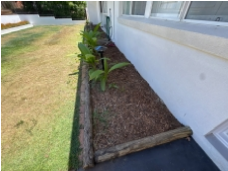
Gardens up against the house hinder the visual inspection zone's, hard surfaces abutting the building are always recommended. A pest controller should be engaged for further assessment.
