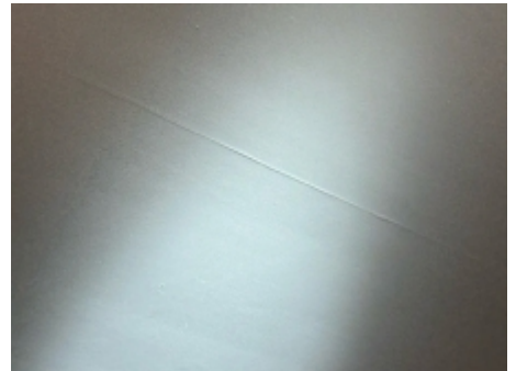
Ceiling cracking was observed, the installation of an expansion joint will reduce the likelihood of this recurring once repaired.
